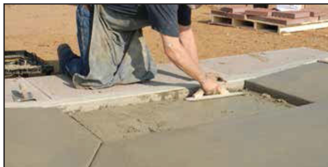
7) Pull out frame. Bull float area to receive detectable warning pavers.
