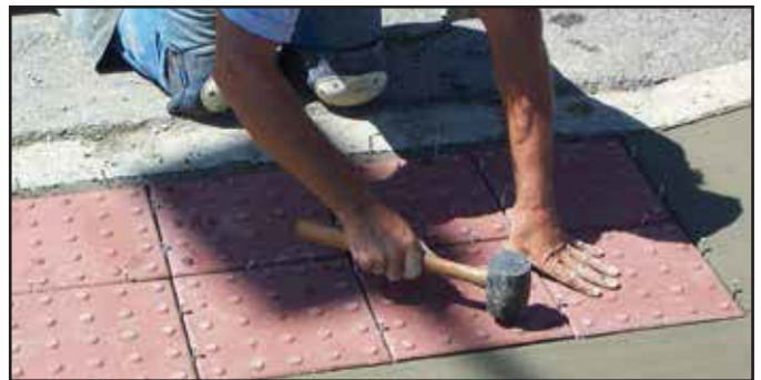
Step #2 - Wet Set Installation - Level pavers by tapping with rubber hammer. Note: Joints may or may not be grouted; contractor option.
