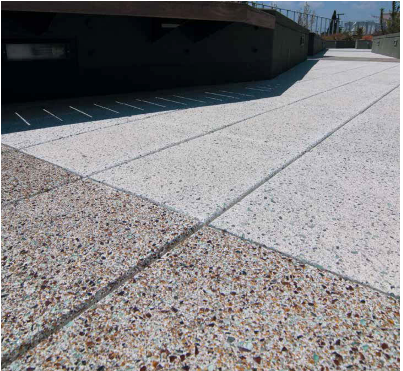
South Los Angeles City Hall, Los Angeles, CA
