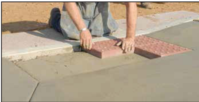
Step #1 - Wet Set Installation - While concrete is still wet, embed pavers into cavity.
