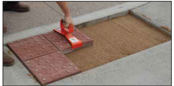
Step #4 - Sand Set Installation - Set pavers in sand. Leave 1/16" to 1/8" between units to allow for sand.
