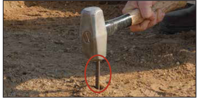
2) Drive in rebar to the approximate height to receive Wausau Tile's block out frame. The frame work has small feet to help locate where rebar should be located.
