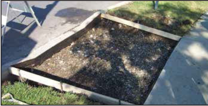
1) Prepare area to receive concrete and detectable warning pavers.
