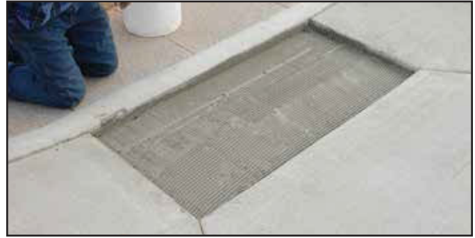
Step #2 - Thin Set Installation - Spread fully and evenly.
