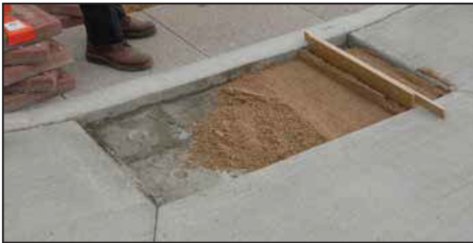
Step #3 - Sand Set Installation - Screed 1/4" masonry sand.
