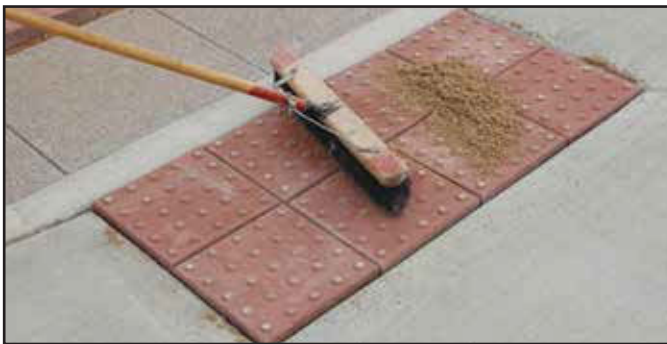
Step #5 - Sand Set Installation - Sweep sand into joints after installation.
