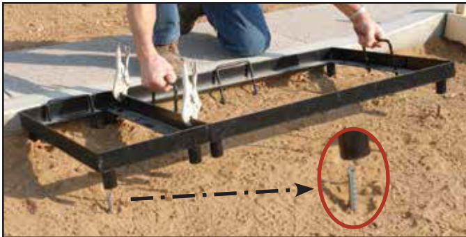
3) Set block-out frame so rebar sits inside the frame legs.
