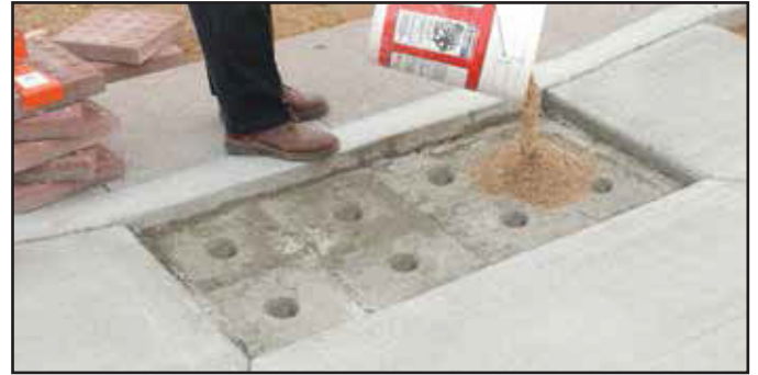
Step #2 - Sand Set Installation - Add masonry sand to recessed area.
